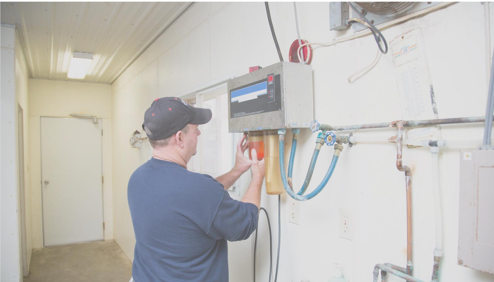
The installation of a refrigeration heat recovery (RHR) unit provides one of the fastest paybacks on a dairy farm. This unit captures the heat from the refrigeration system to preheat well water up to 140 degrees, while also improving the efficiency of your refrigeration system. Major advantages to installing an RHR unit include:
